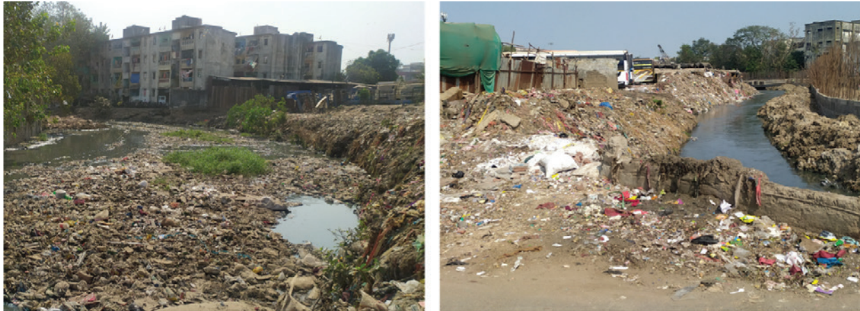
Figure 26. Example of waste disposal in waterways canals
