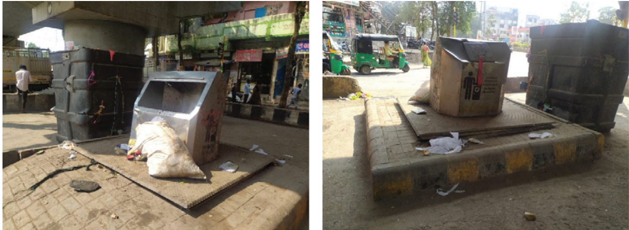
Figure 16: Front (left) and back (right) of underground smart dustbins
