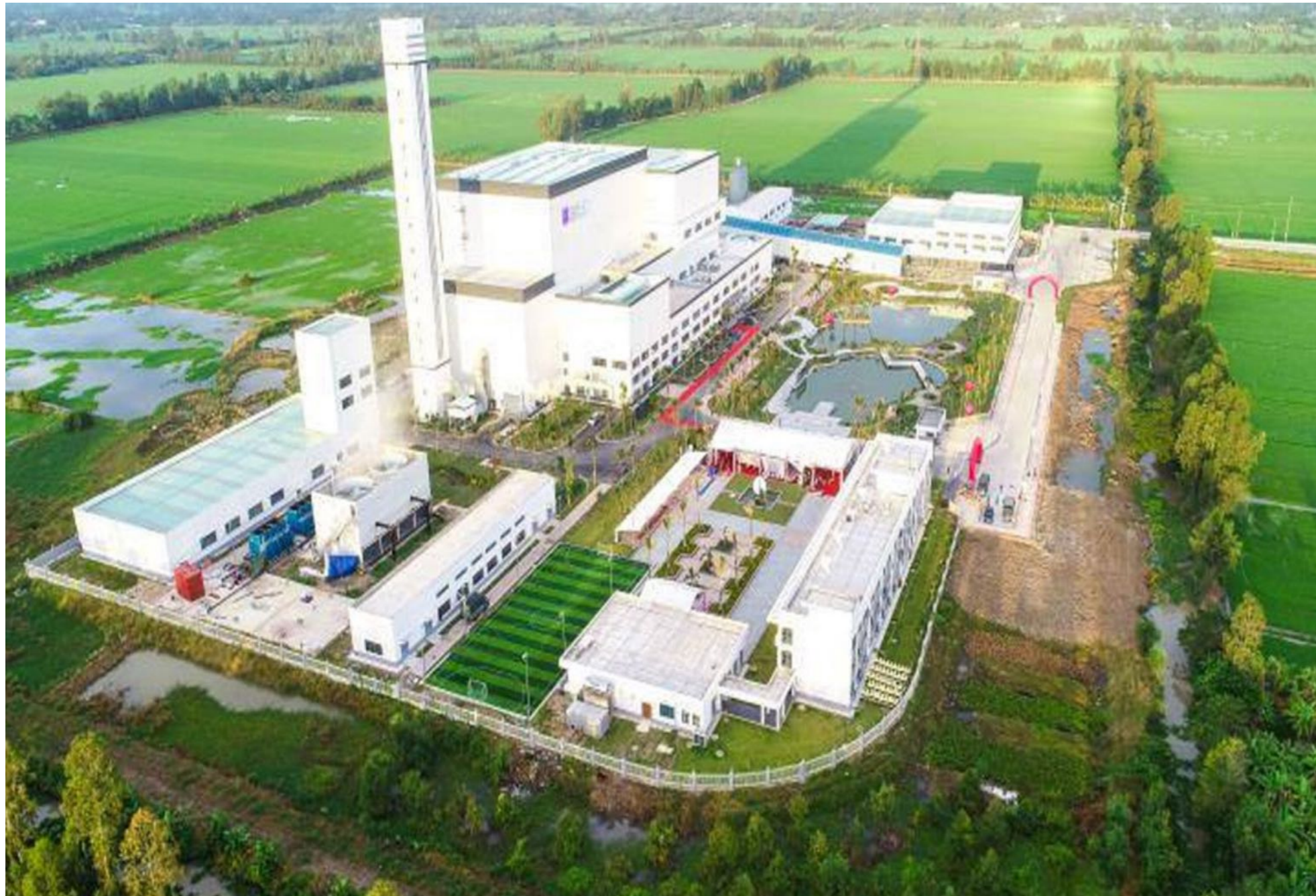
Can Tho waste-to-power plant
